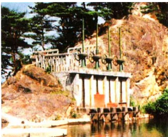
Former Kaduma Anazeki Headworks
