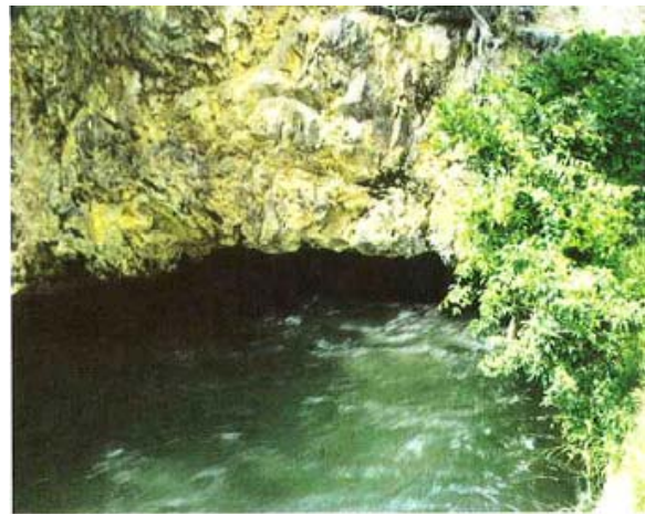
Water intake at the former Kaduma Anazeki Headworks
