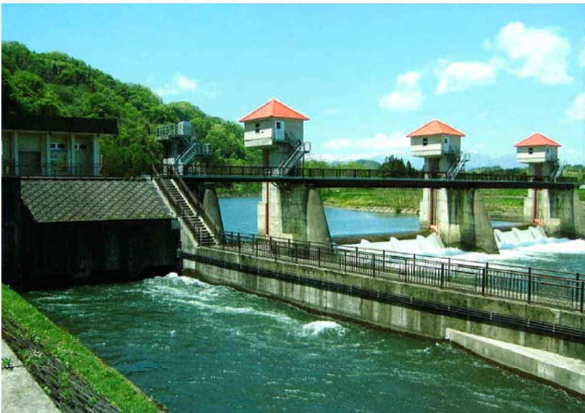
Kaduma Anazeki Headworks
