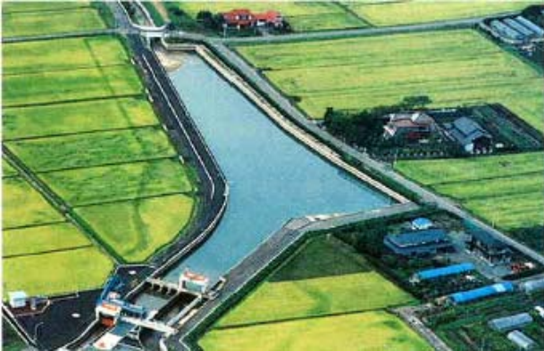
Inariba Large Diversion Work
